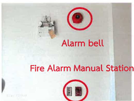
Alarm bell & Fire Alarm Manual Station
