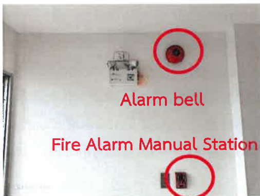
Alarm bell & Fire Alarm Manual Station
